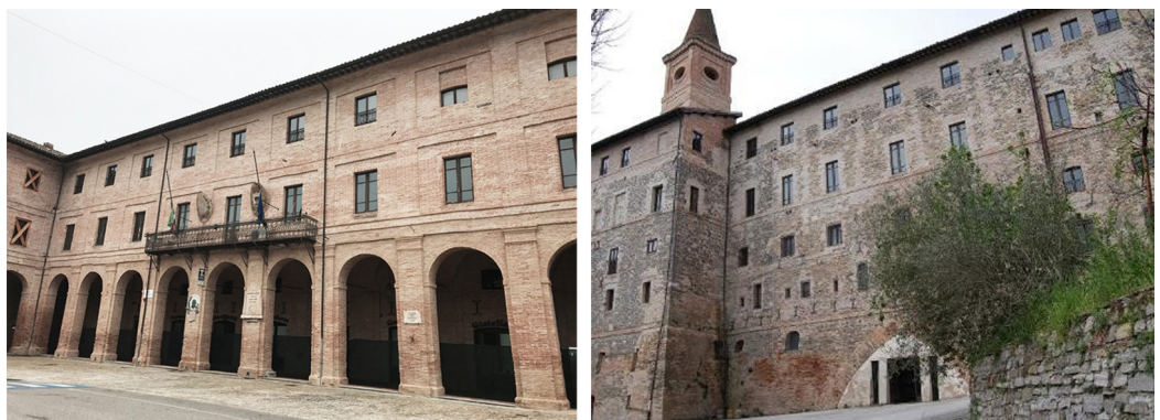
Fig. 01. Photographs of the exterior elevations show the clear break between the main front and the back side of the building. Photo by the authors (2021).
