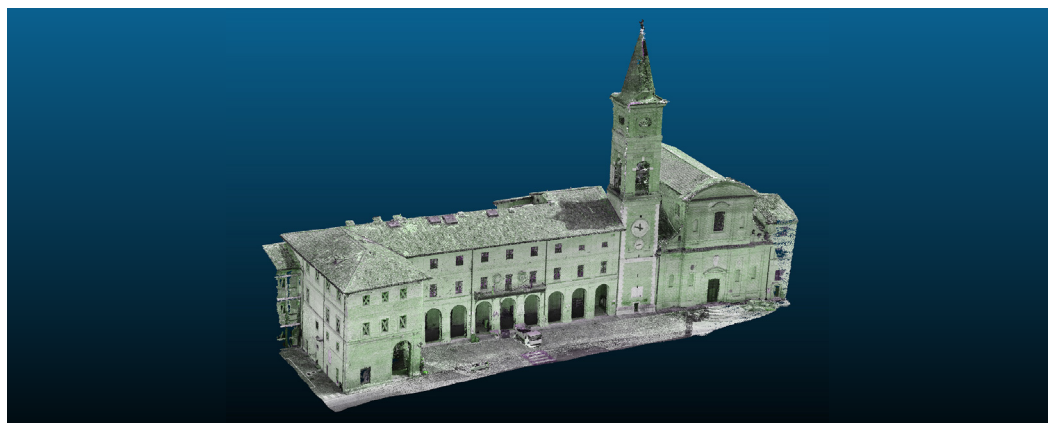
Perspective visualisation of the point cloud of Palazzo Pallotta in Caldarola. Image processed by the authors.
